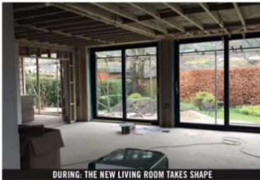
DURING: THE NEW LIVING ROOM TAKES SHAPE
