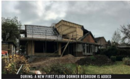
DURING: A NEW FIRST FLOOR DORMER BEDROOM IS ADDED
