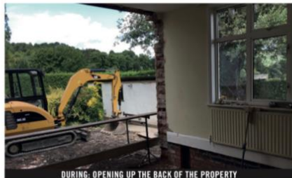
DURING: OPENING UP THE BACK OF THE PROPERTY
