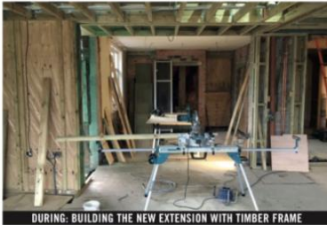
DURING: BUILDING THE NEW EXTENSION WITH TIMBER FRAME
