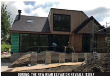
DURING: THE NEW REAR ELEVATION REVEALS ITSELF
