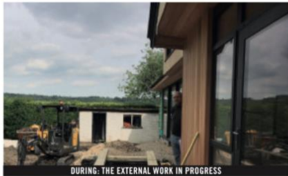
DURING: THE EXTERNAL WORK IN PROGRESS
